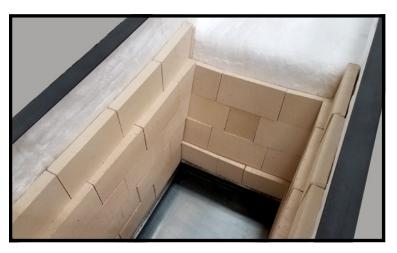
Finished bricking. Side wall and ramp of the firebox.
