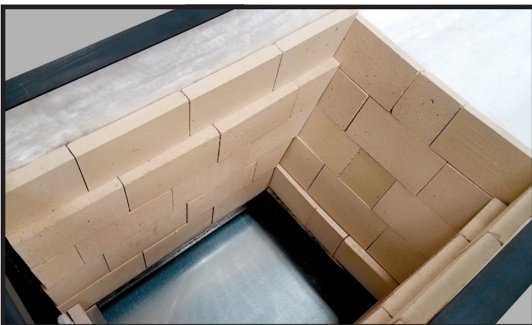
Finished bricking. Side wall and ramp of the firebox.
