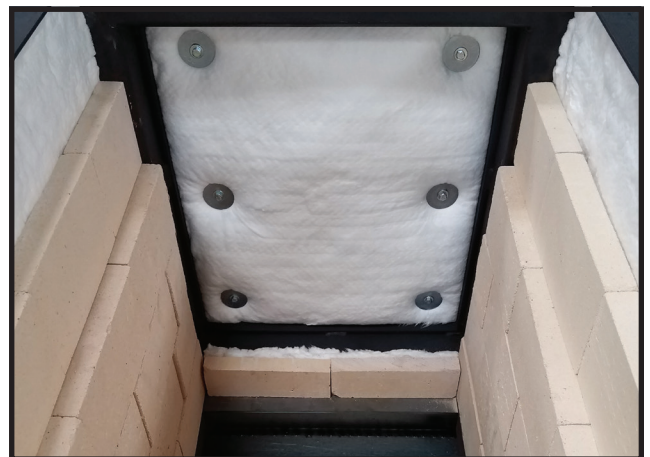
Finished bricking. Backside of the front door frame.
